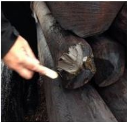
Using the disposable spatula distribute the putty over the surface approx 3mm
