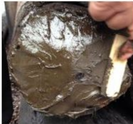
Using the disposable spatula distribute the putty over the surface approx 3mm
