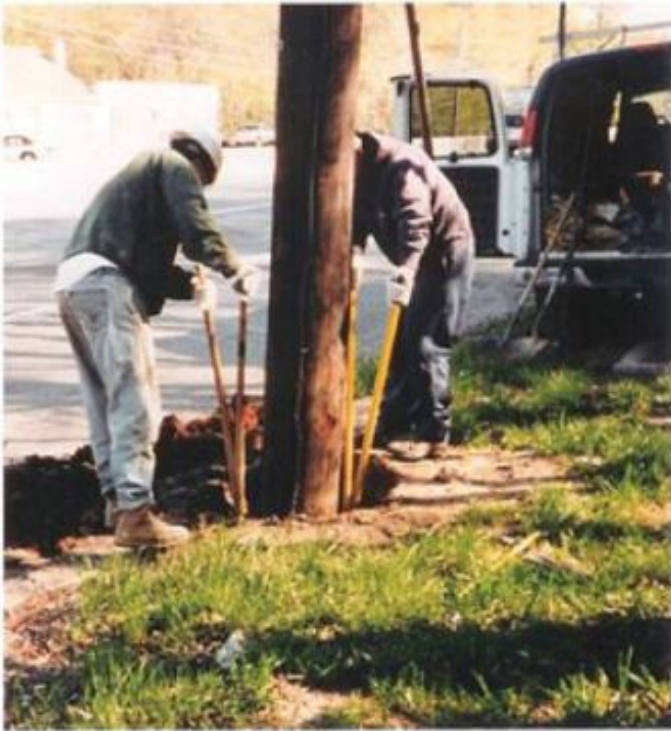
Excavate around the pole to a depth of 0.7m
